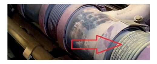
Calcium chromate particles are detected on more and more turbines and engines during service work after the insulation systems that have been in use have been uninstalled. The deposits are not only found on the previously insulated objects, but also on the inside of the insulation material.
